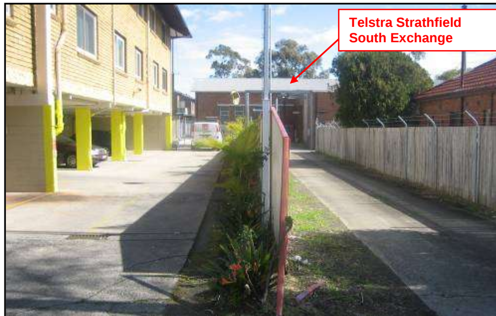
Figure 6: View of the vehicular access way to the Spanish Motor Inn site.
