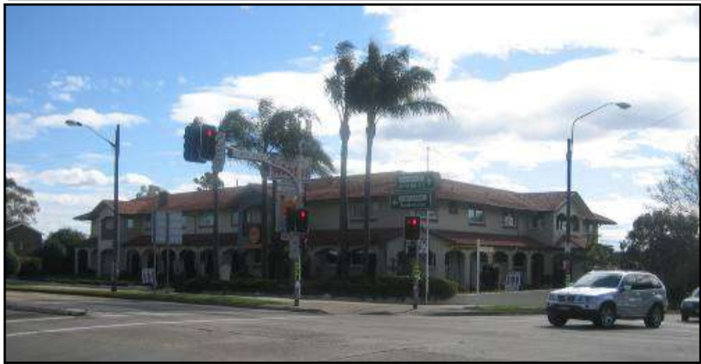
Figure 4: The Spanish Motor Inn as viewed from the intersection of Liverpool and Homebush Roads.
