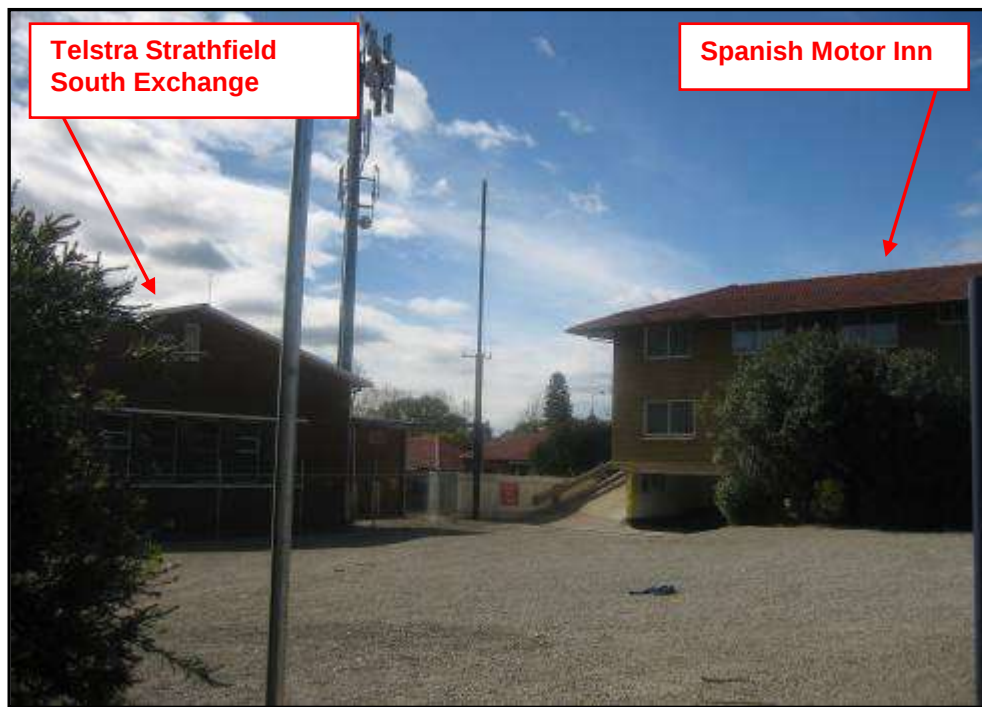
Figure 5: The Subject Site detailing the relationship with the Telstra Exchange and the vacant site to the west
